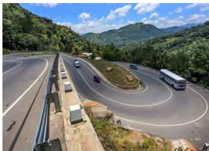
The Kandy–Mahiyangana national highway in central Sri Lanka was upgraded under the ADB-supported National Highways Sector Project.
