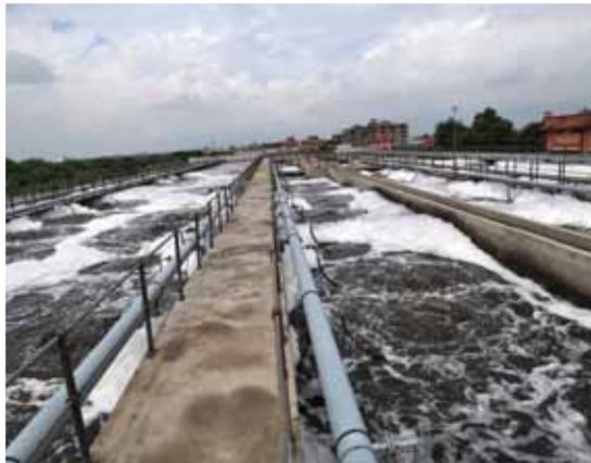
The Delawas Sewerage Treatment Plant, built in Sanganeer, Rajasthan, under RUIDP-I, treats about 62.5 mld of effluent and sewage generated by Jaipur City
