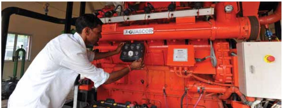
The methane tapped from the Delawas STP is used to generate clean electricity to run the entire plant
