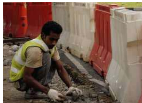
A foreign laborer works on a construction project in Singapore.
