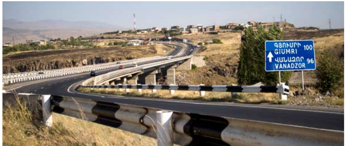
The Yerevan–Gyumri highway is part of the North–South Road Corridor.
