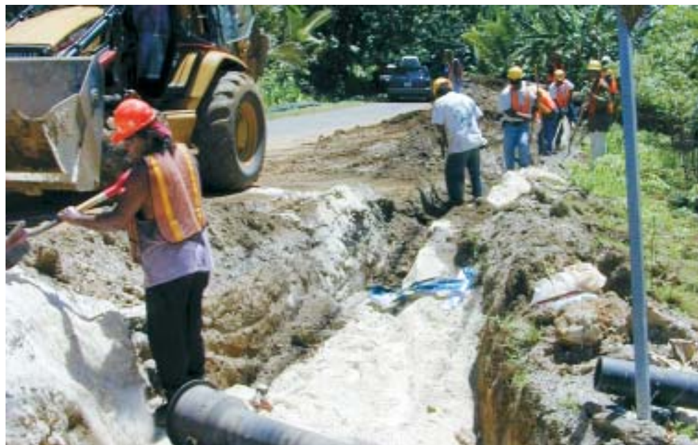
Workers lay down water pipes in Pohnpei.
