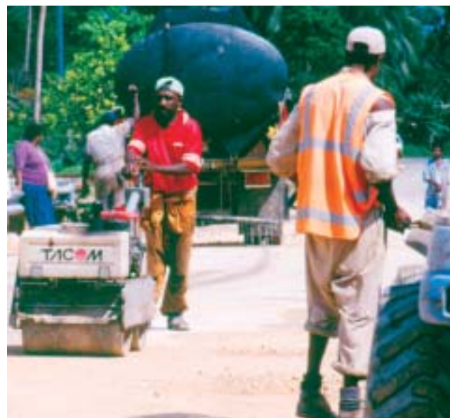
ADB-funded road construction.
