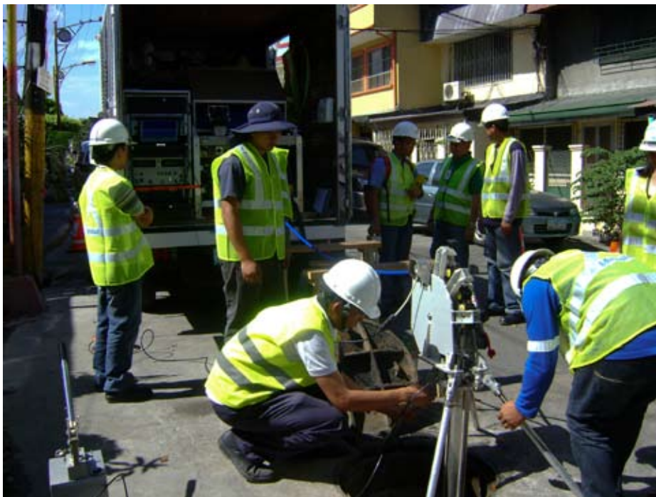
Trunk main inspection in Manila
